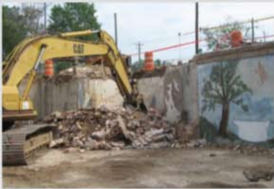
LRADAC Testing and Demolition Project
