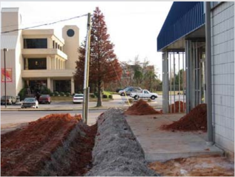
Dennis Corporation performed Building Construction Management for their new corporate headquarters
