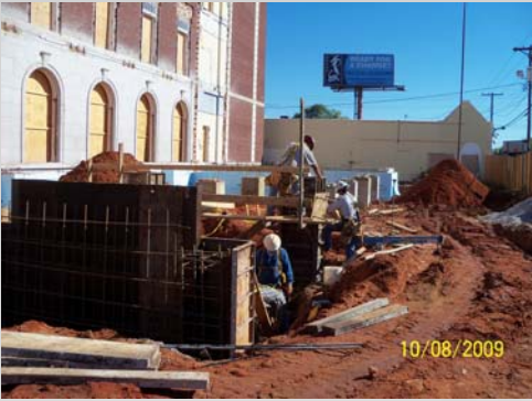
Reinforcement and formwork for foundation walls at the Township Auditorium
