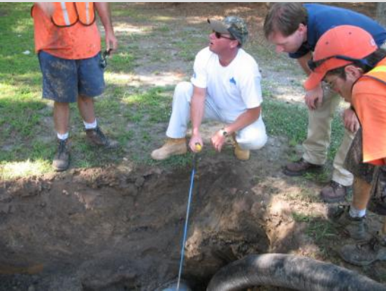
Dennis Corporation Staff at Pipe Inspection
