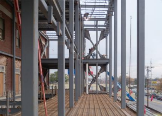
Steel Frame Construction
