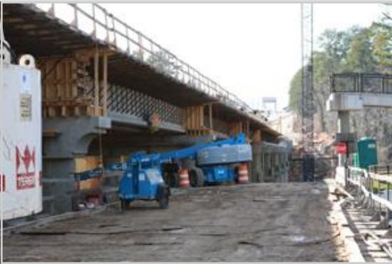
Broad River Road Bridge Project
